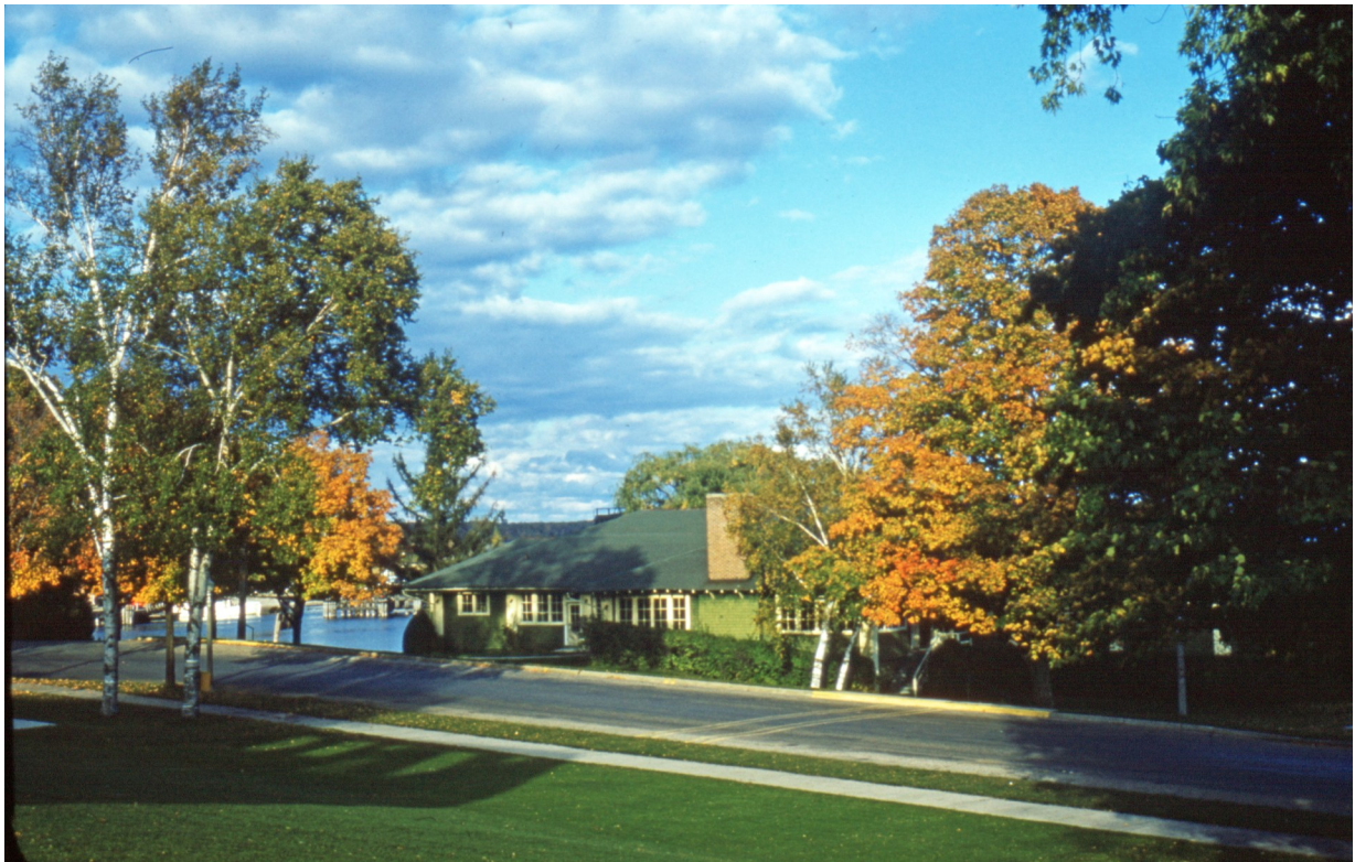
View northeast over Ferry Avenue. Only the chimney remains standing.
