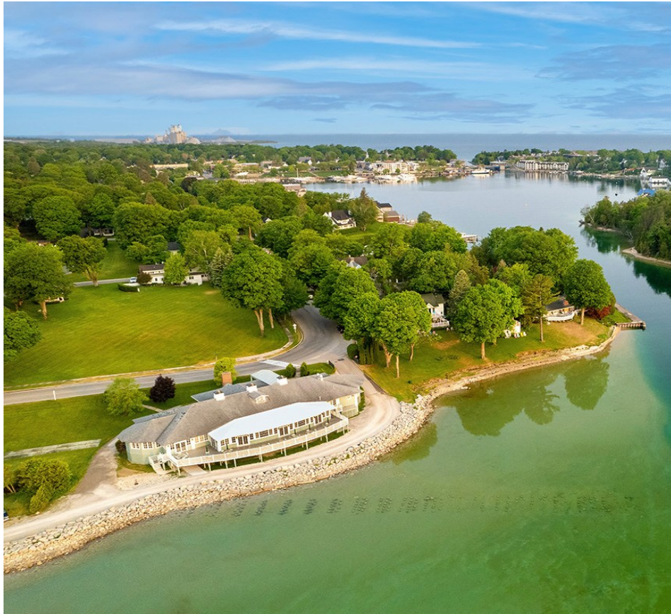
Before, June 7, 2023, showing added exterior viewing balcony .
