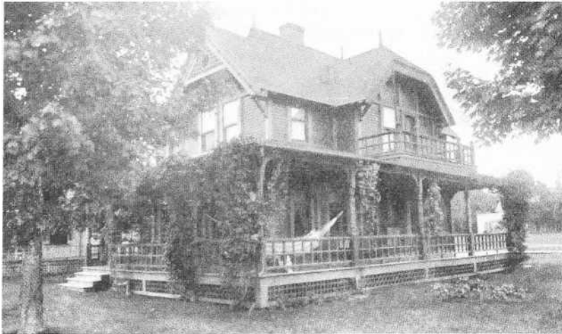
First cottage on the Belvedere — northeast view — present owner Bill Eberts, cottage No. 111, 1900's.
