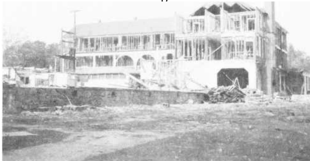
And the walls came tumbling down, September, 1960.
