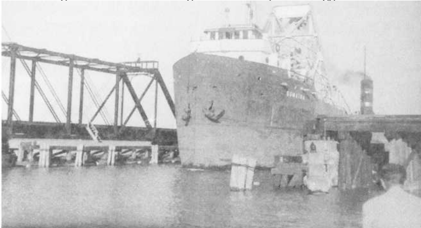
The coal boat Sumatra coming through the channel. That year she knocked out the south end of the trestle, making the bridge inoperable, 1946.
